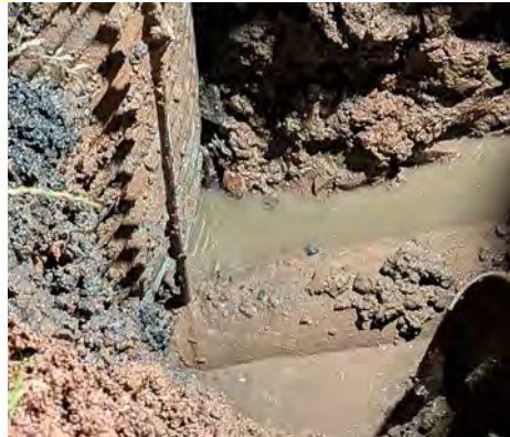
Damage to the pipe called for immediate action. Here you can see the leak.
